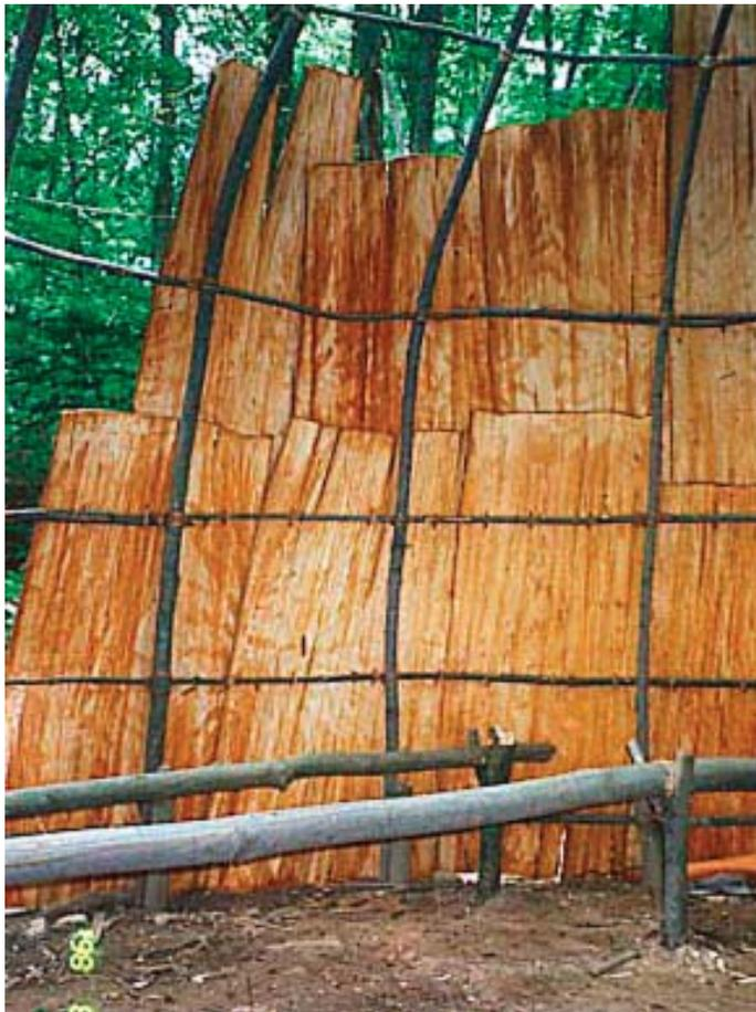
**Fig. 9** External poles are used to secure the bark to the inner framework
