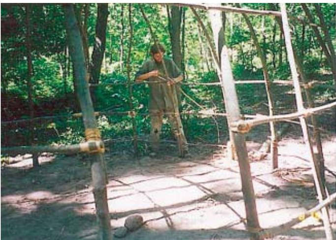
**Fig. 4 Horizontal rings added to the vertical arches for additional strength**
