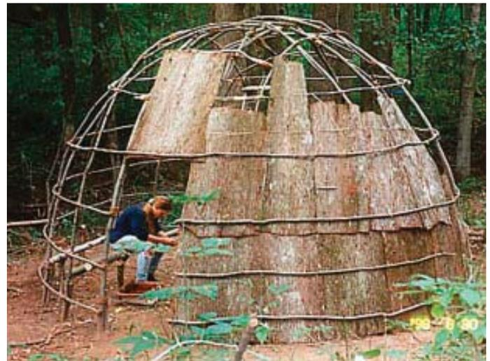
**Fig. 10** Note the spruce root clamps at regular intervals along the lower two rungs
